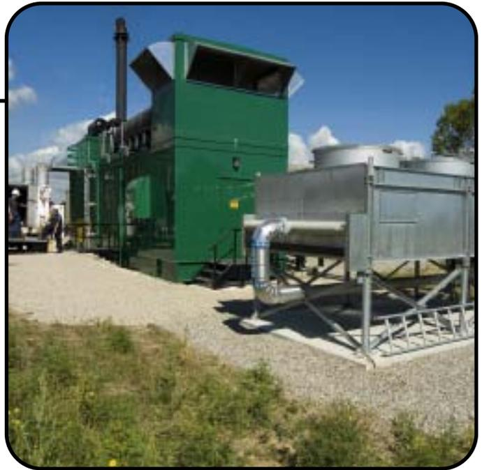
Toromont Power Systems installed this turnkey 1.6 MW digester-gas-fueled cogeneration system at the Woodward Avenue Wastewater Treatment Plant in Hamilton, Ont. It's powered by a Cat® G3520C gas engine configured for low-energy fuel.
